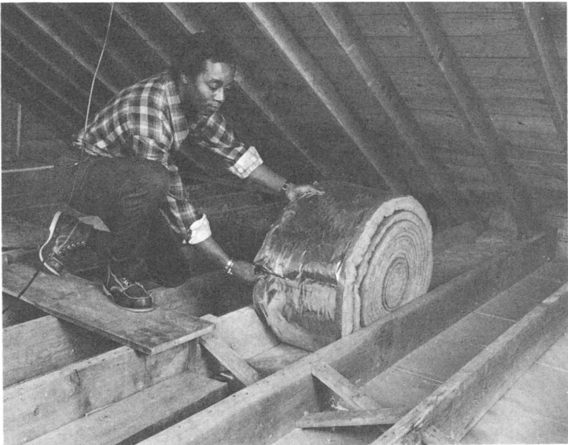
Insulating the attic of a house.
